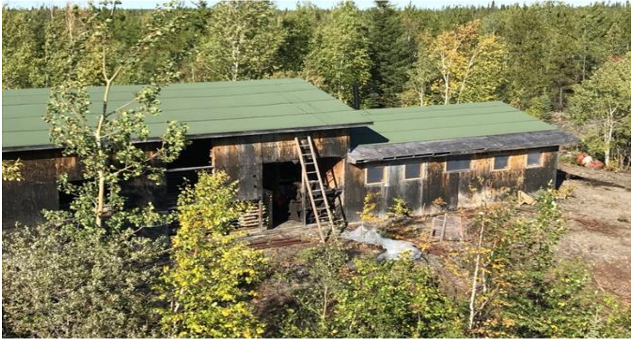
Figure 32: Building used for core logging and core storage at Lingman Lake
