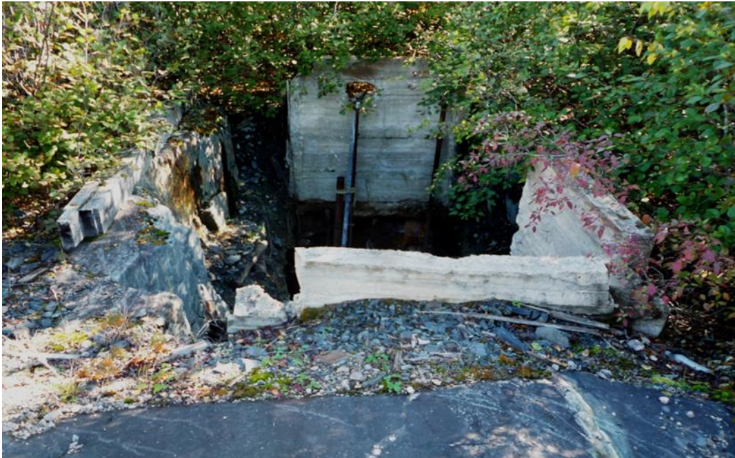
Figure 39: Shaft collar looking east.
