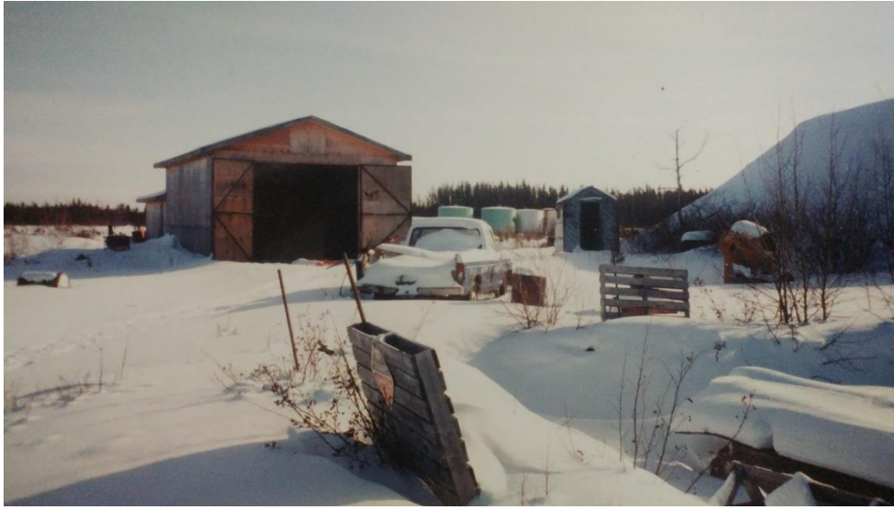
Figure 10: Garage building now used as core logging facility, photo 1990
